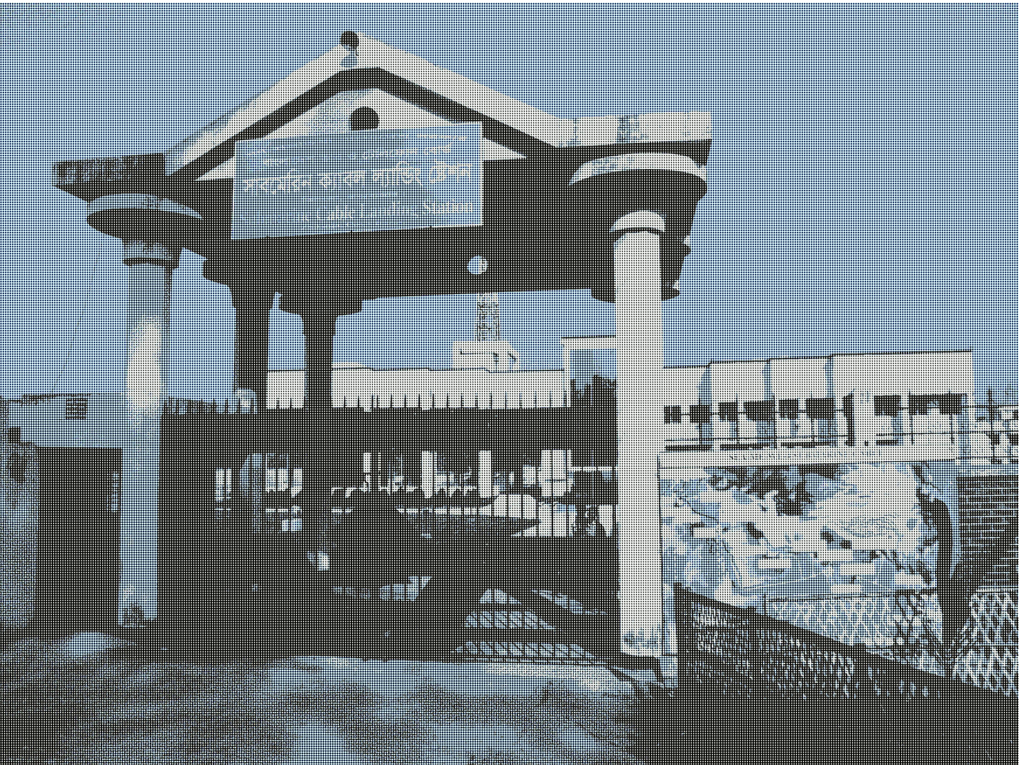
Figure 4. Submarine cable landing site, Cox's Bazaar, Bangladesh (2006)
